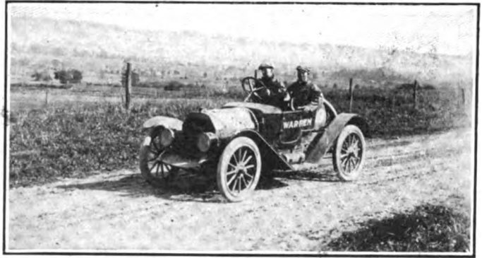
Warren finishing third day's run through the hill country
